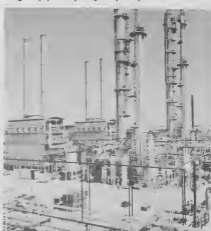
Completed Hydrogen Plants north of Powerhouse No. 1. Plantas Hidrogeno completa, noord di Powerhouse 1.
